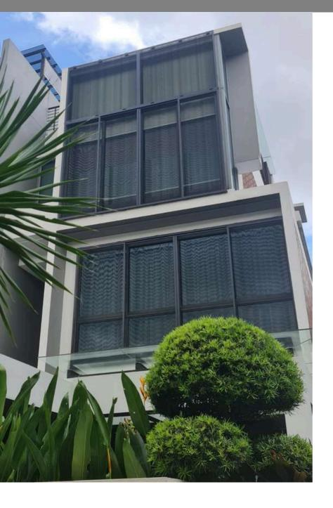
In order for glare to be eliminated, the screens were installed outside, on the roof top terrace as the primary protection.
