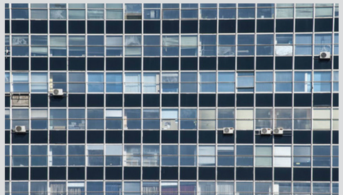
Reality – Internal blinds, lights on and adhoc AC units
