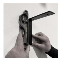
Take one of the shelf brackets and position in the correct location in relation to the wall. Hold the bracket to the wall and using a spirt level, ensure the bracket is vertically level.
