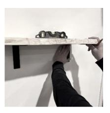
Next, to fix the shelf to the brackets, place the bracket on the shelves in your desired position and draw pencil marks to show where the pilot holes are to be drilled.
