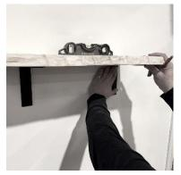
Next, to fix the shelf to the brackets, place the bracket on the shelves in your desired position and draw pencil marks to show where the pilot holes are to be drilled.
