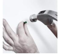
Gently push the provided Rawl plugs into the holes and then screw the bracket onto the wall remembering to drive the screw until the bracket is tight.
