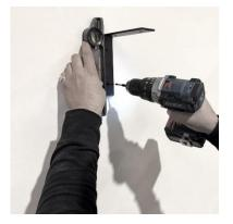
Take the second bracket and position it on the wall in your desired position. Then taking a spirt level, level the tops of the 2 brackets horizontally and then with the bracket you are about to fix, level it vertically. Draw pencil marks to show the location of the bracket holes and then with a 2mm wood drill bit, drill 10mm pilot holes. Screw the provided fixings into the pilot holes and secure the bracket.
