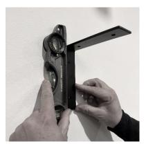
First find the timber studs using a stud finder and while timber stud fixing widths can vary, they are usually spaced at 400mm. Take one of the shelf brackets and position in the correct location in relation to the wall. Hold the bracket to the wall and using a spirt level, ensure the bracket is vertically level.
